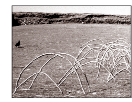
Pre-bending hazel rods to form the ribs of a Donegal curach. c.1910 35
