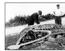
Later, a boulder holds down the stem while it is built upside down
