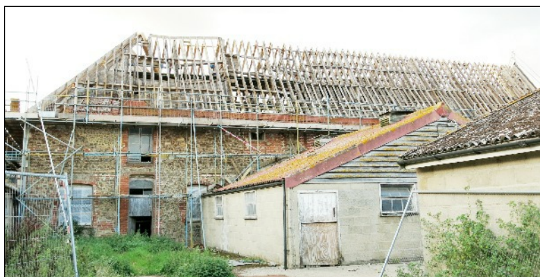
(left): Kitchen doorway with 16th century window opening and fireplace; (right) Kitchen ceiling beams with boarded loft above; (below) south elevation during restoration of the roof. The door will have opened into a kitchen yard.
