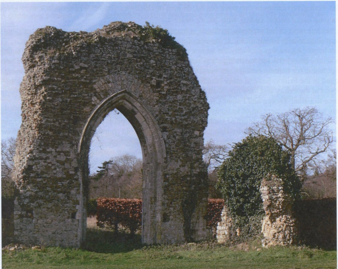
The south transept arch of the Priory church, one of the few fragments, apart from the fine Gatehouse, still standing (photo Richard Quarrell)
