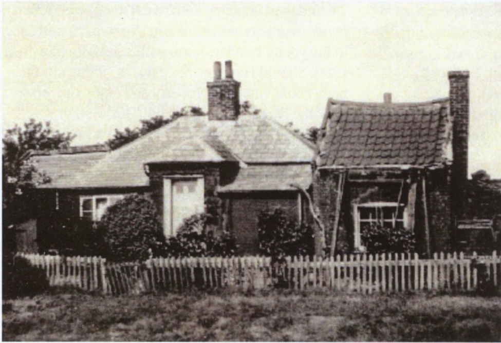
The dilapidated building in front of Dennington Cottage likely to have been used by signalmen (Orford & District Local History Bulletin: Issue 31)
